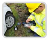
The Cello 6 Meter Reader uses the existing highly developed and regularly maintained GSM SMS / GPRS communications network to transmit indices (meter readings) and consumption profiles to a host server at user defined intervals. Meter readings and profile data may be sent to either Technolog's own proprietary software 'PMAC Plus' or an Oracle based server for export into an utilities own billing system.
