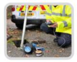
The Cello 4 is a fully integrated wireless data logger. It has two digital / flow inputs with optional internal pressure, PRV control, state / pump duty monitoring and waterfall.
